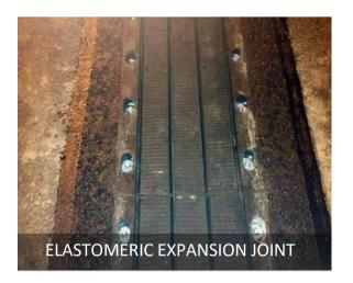
c. Elastomeric Expansion Joint
